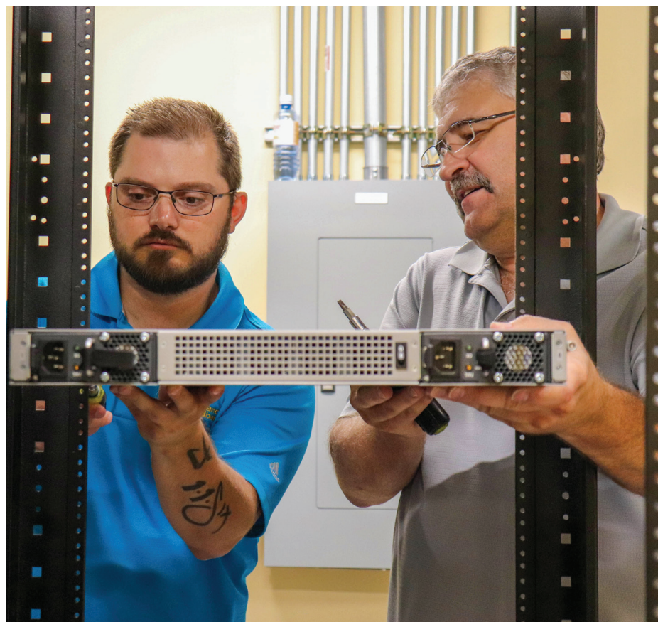
Michael Doyle, IT support technician, (left), installs a router inside a server room with the assistance of Jim Zorn, manager of IT/SCADA (right).
