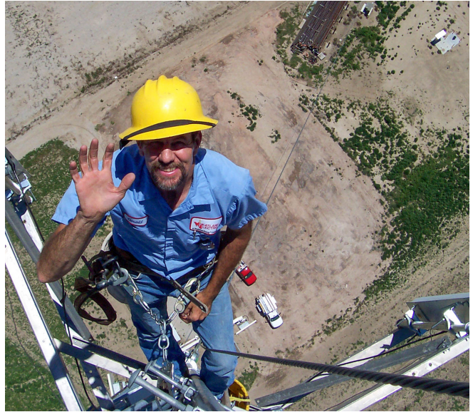
Gearold Leverett inspects coax connections at the top of this 400-foot-high tower in Finney County. Photo circa 2003-2004.
