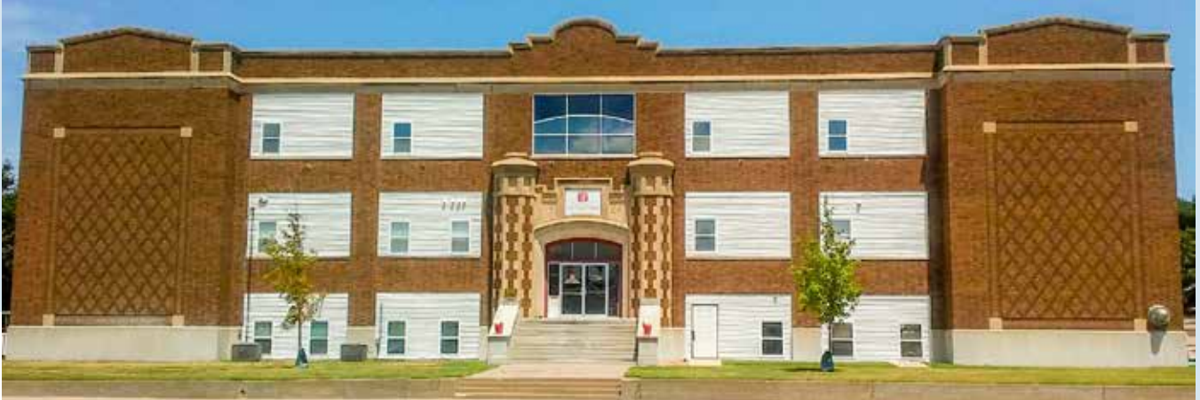
The Central Kansas Dream Center building, located at 2100 Broadway Avenue in Great Bend.
