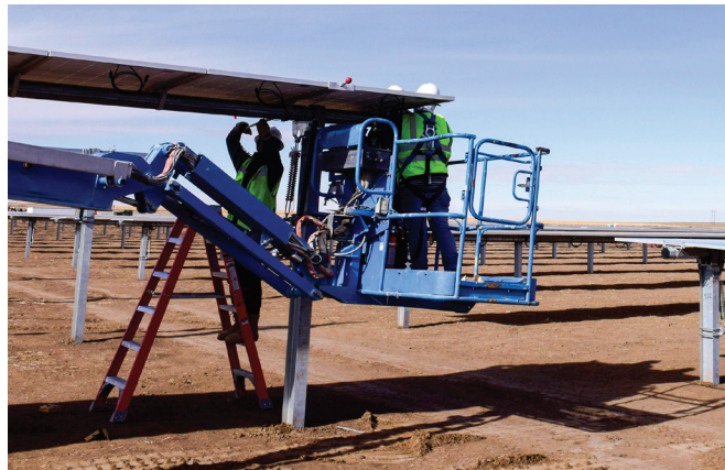
For Johnson Corner Solar Project to generate 20 megawatts crews installed 75,012 solar panels.
