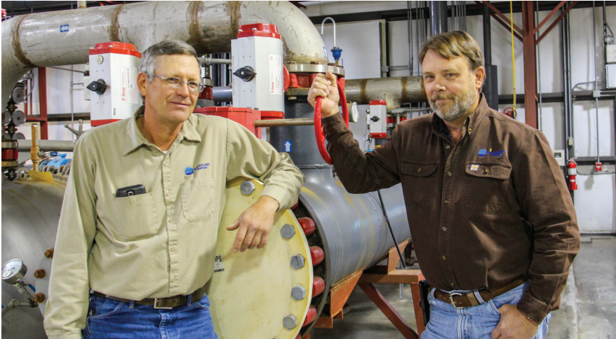
Francis Lobmeyer, Water Works Technician, and Perry Smith, Manager of Water Works, stand at the 20 inch incoming raw water pipeline that feeds the reverse osmosis skids. Air operated valves (red valves) are mounted on the piping and function when the plant is called to run.
