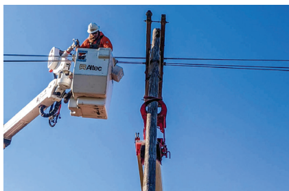
Brandon Ritchie, journeyman lineman from Great Bend, works to restore power in and around Pawnee County. Wheatland sent a line crew to assist Midwest Energy Inc. during widespread outages in late March.
