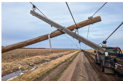
During severe weather, line crews act as safely and quickly as possible to begin restoration. Never approach downed power lines and contact Wheatland Electric or first responders immediately if you see them.
