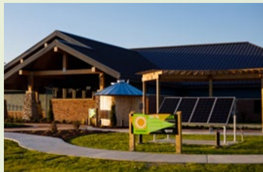
Great Bend's outdoor green space features off-grid solar panels, a corrugated steel rainwater tank, and an air turbine.
