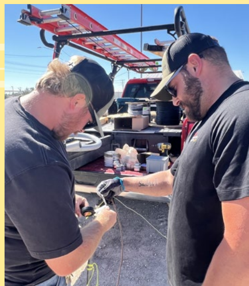
Cory Eli (right) and Taylor Heili, both wireless tower technicians, organize and connect wiring for a card security reader at WEC’s Leoti office.
