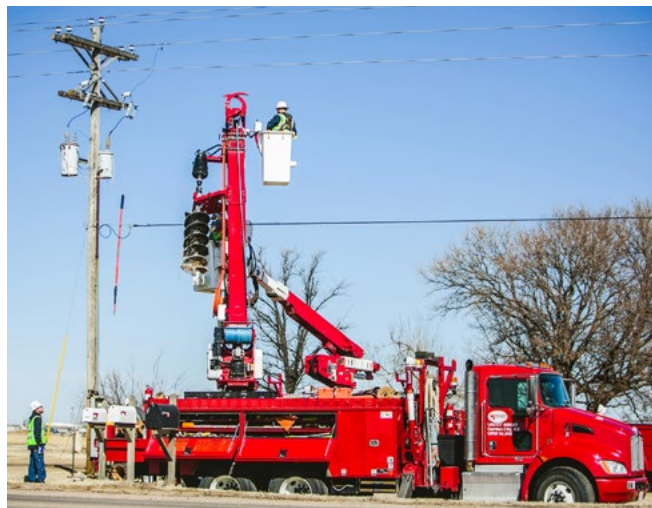
A WEC lineman works from an aerial bucket while another crew member assists from the ground during infrastructure improvements in Finney County.
