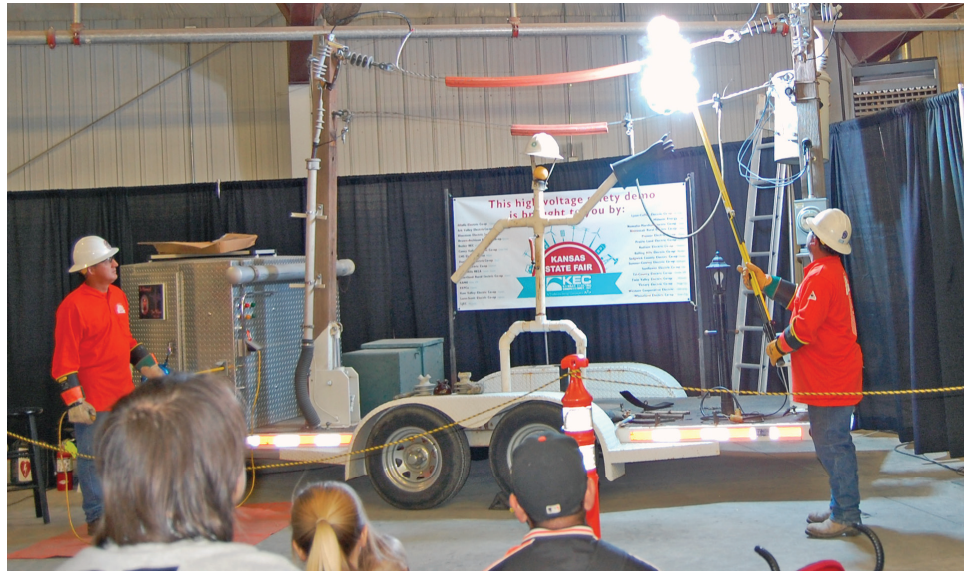
Trent Suchy (right) and Matt Hosler, both Substation Technicians from Great Bend, conduct the high-voltage demonstration.
